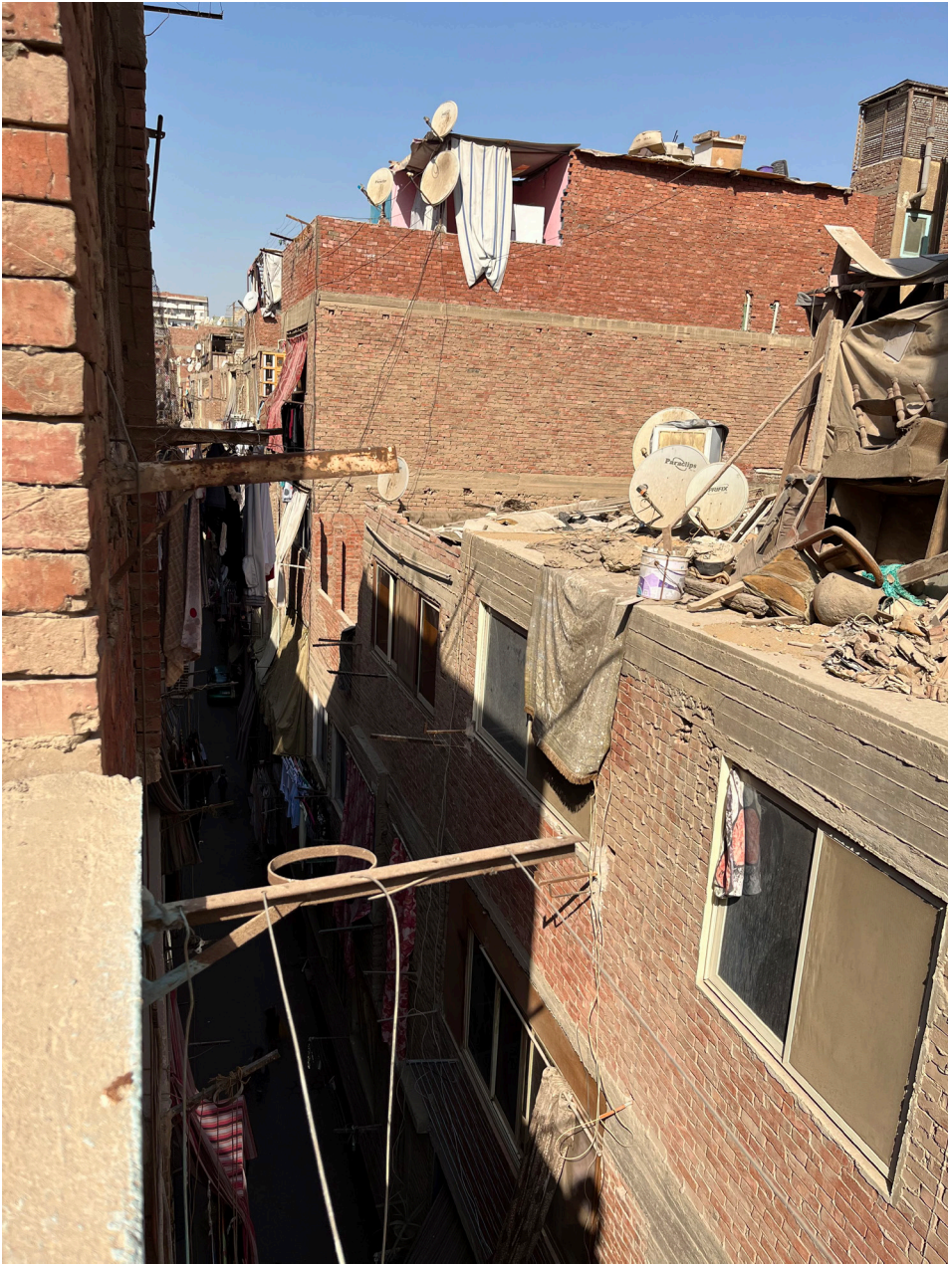
Context: the Phase 2 of the workshop focused on the spatial transformation of a community school for Sudanese refugees in the informal settlement of Boulak Al Dakrour, Cairo.
